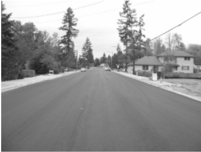
Newly paved 73rd Avenue NE, looking north
