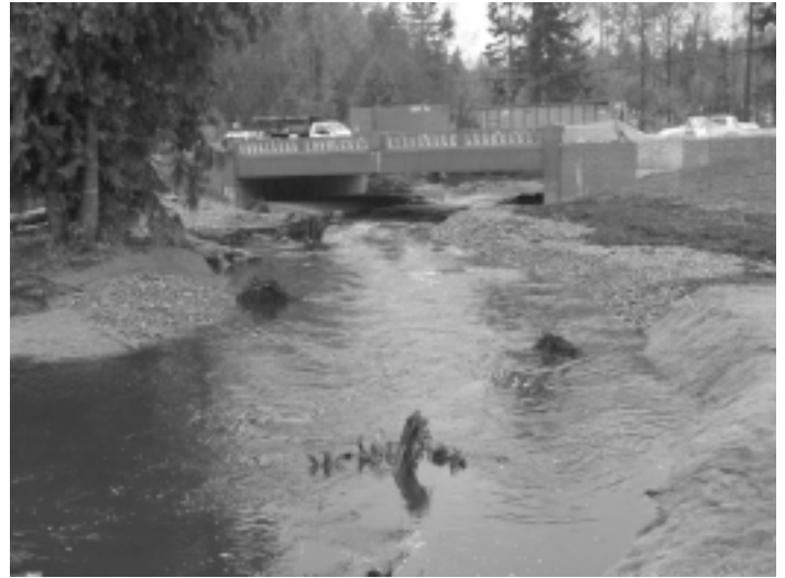
New 73rd Avenue NE Bridge over Swamp Creek and new channel
