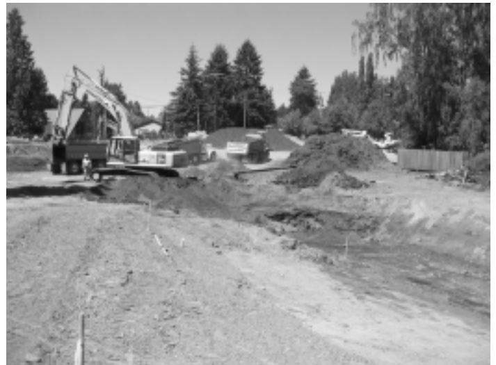
Excavation of new Swamp Creek channel
